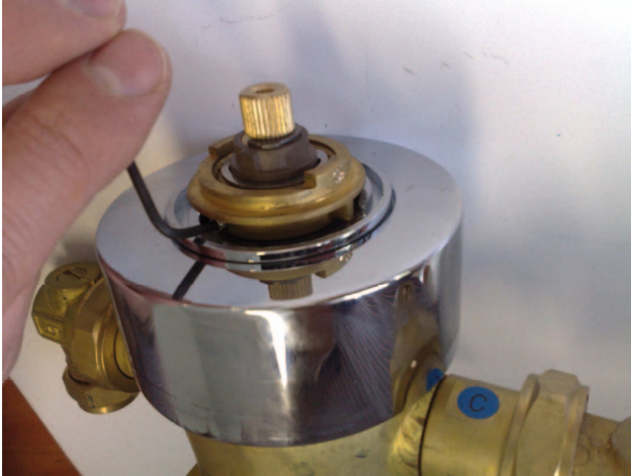
1.5 Remove the brass fixing collar.
