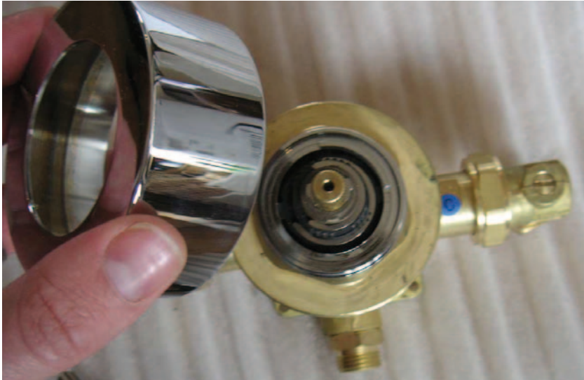
1.7 Remove the body cover ring by turning anti-clockwise
